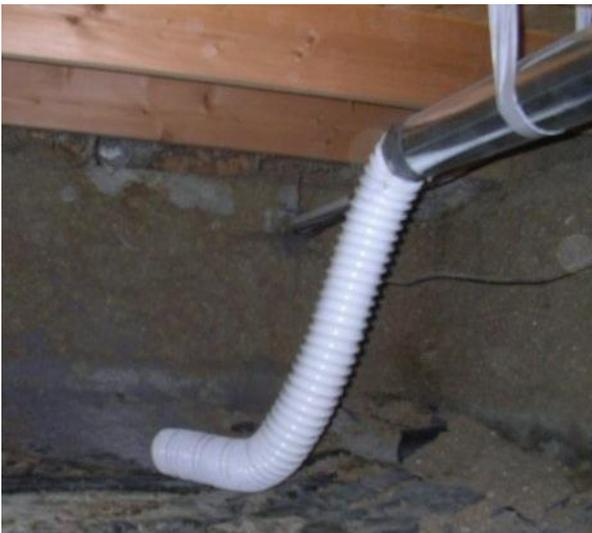
Providing gentle curves, such as a pair of 45° elbows, instead of 90° elbows, improves the flow when changing direction. Checking the location where the exhaust vents exit is also important, because exterior obstructions can reduce the flow.
