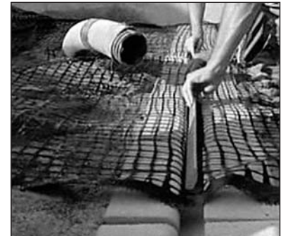
Lock bar installation
