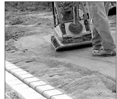
Backfill and compact
