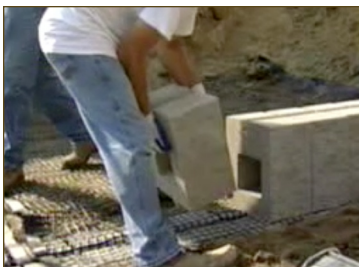
Diagram 5—Full Unit Installation
