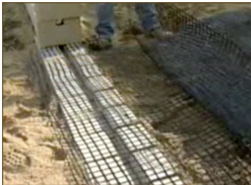
Diagram 9—Geosynthetic Reinforcement
