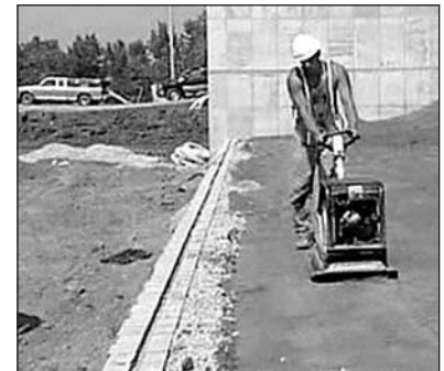
Backfill and compact
