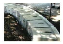
Top block (pictured right) may not be appropriate for all situations. A 6" recess in the top of the block allows for backfilling behind the wall. The void allows you to fill up and over the top of your wall. It is deep enough for any landscaping to take root.
